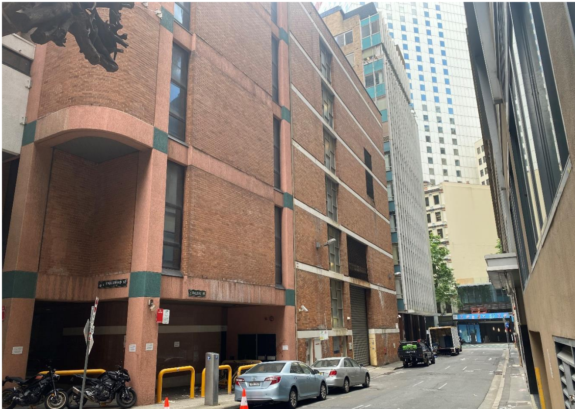
Figure 3: Site viewed from Dalley Street
